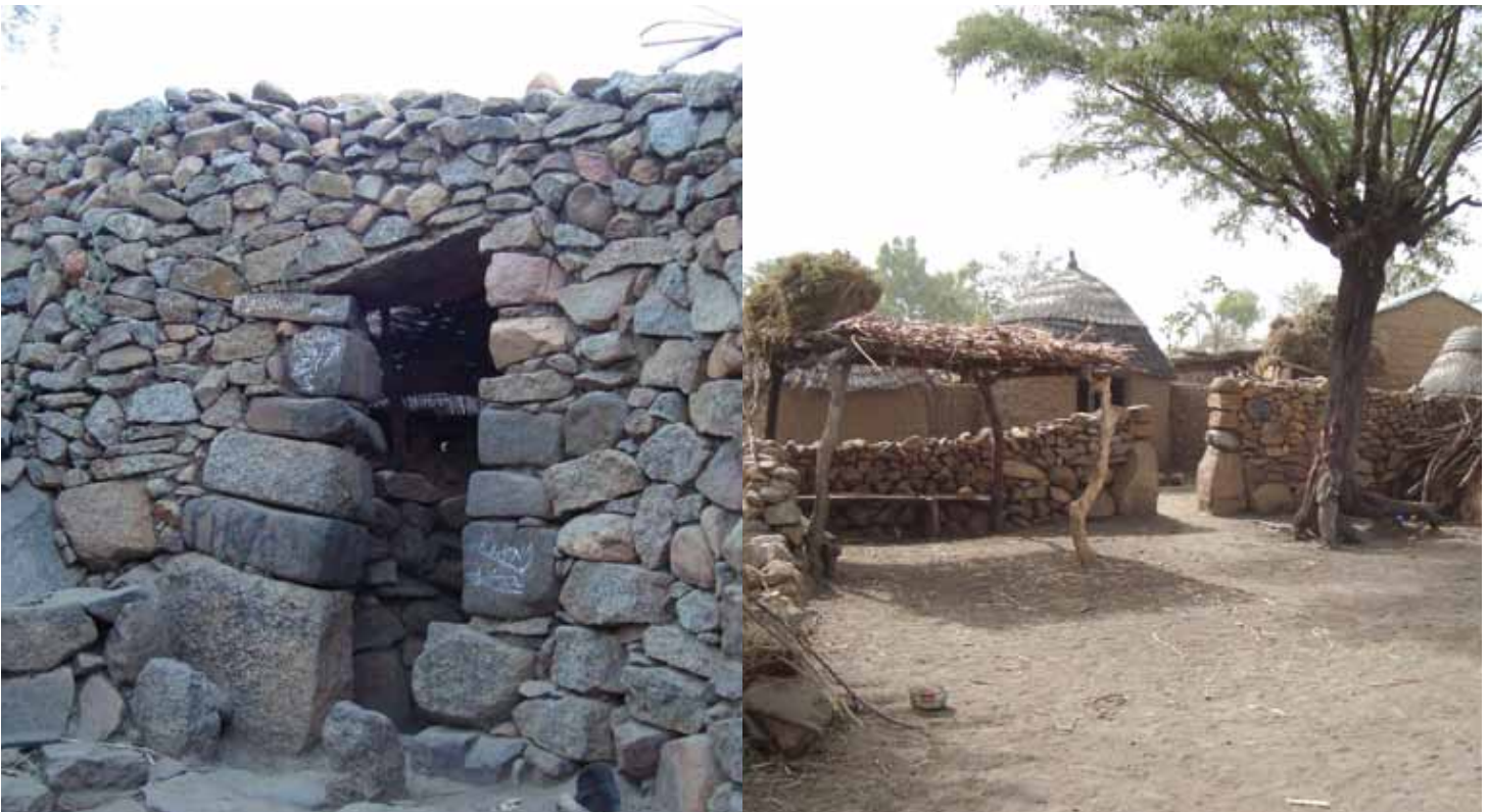
Figure 4: Left: a stone lintel over the entrance door of the residence of a Sakun leader. Right: the entrance of a typical Sakun residence with no lintel. © I. Odiaua
