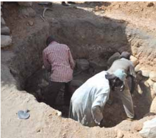
Figure 6: Construction of a sub-basement bullpen. © Michael Thomas
