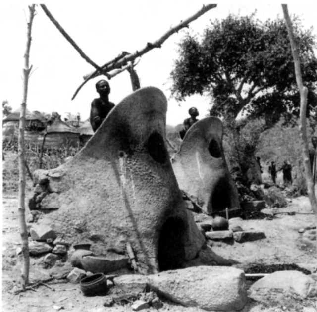
Figure 2 (below): Teleki furnaces, estimated height c2m. According to Gardi the men are singing and pumping the bellows, but it is far from clear that a smelt is in progress (Gardi 1953, Plate 54). Photo René Gardi 1953/77/12 by kind permission of Bernhard Gardi.
