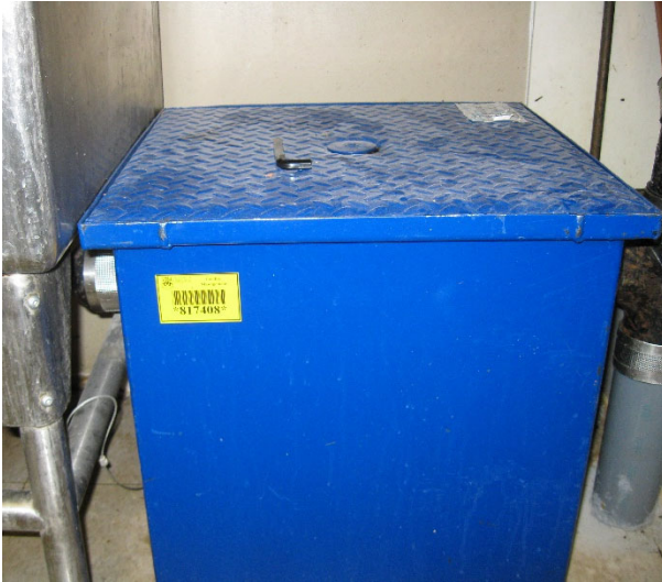
Example 9. Grease Interceptor
